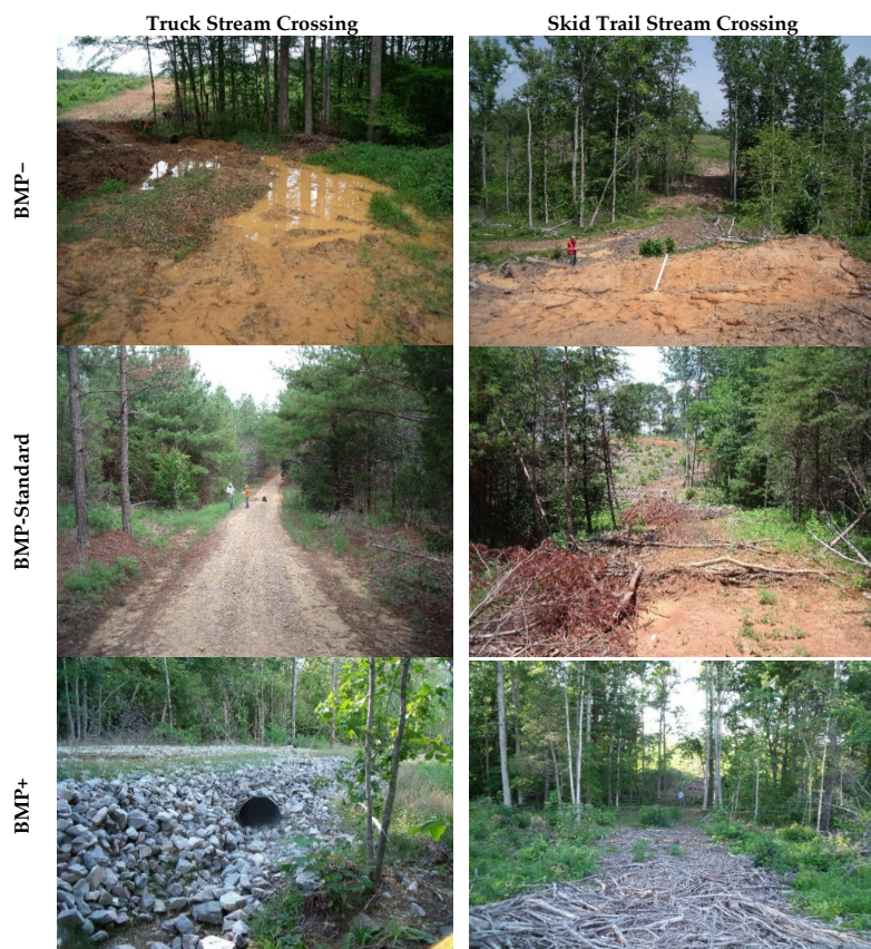
Figure 3. Representative photographs of the three BMP levels for the two crossing types.
